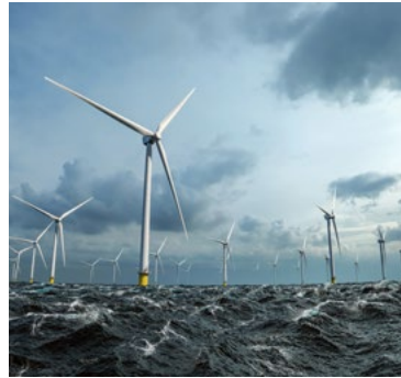
Offshore wind power
