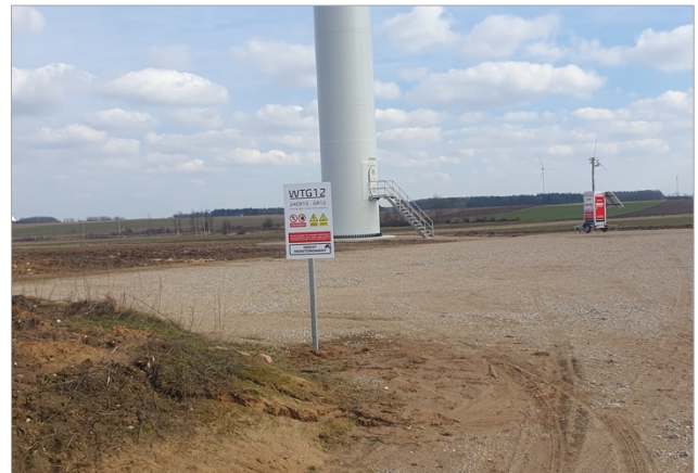
Photo 7.2 Warning sign placed in the vicinity of WTG12
