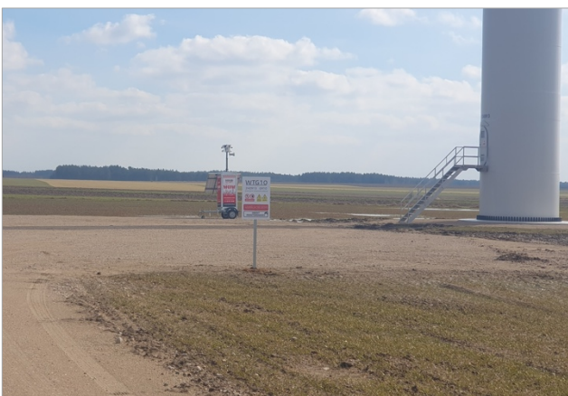
Photo 7.3 Warning sign placed in the vicinity of WTG10
