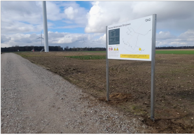
Photo 7.5 Information and warning sign placed at the main entrance to the wind farm
